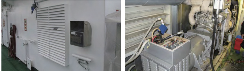
Figure 15.1 Damper of the emergency generator SOURCE Investigation report(AIBN)
