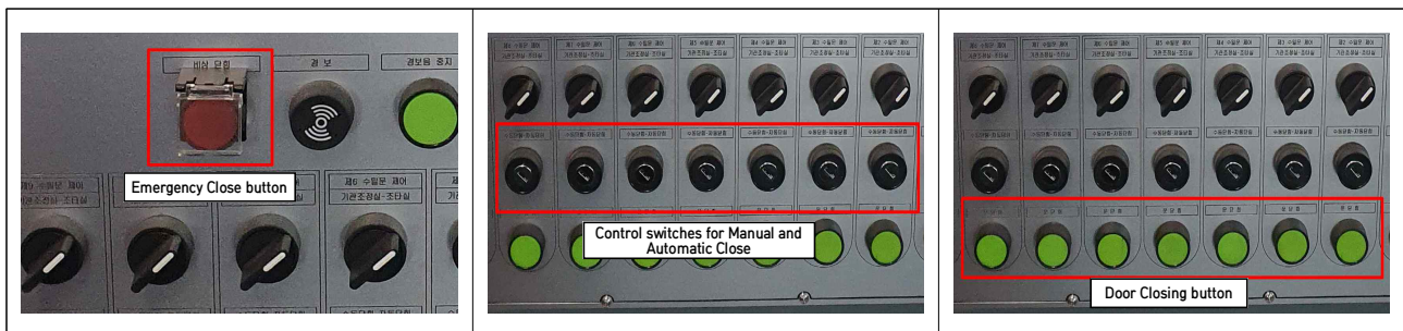
<Figure 17> "Emergency close" button (left); "automatic close" switch (middle); and "door closing" button (right)
